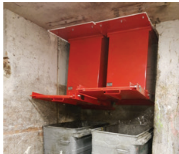
A 240 min fire-rated chute discharge pipe/chute extension is required when no fitting directly to the FCP directly to the ceiling slab. (Illustrated)
